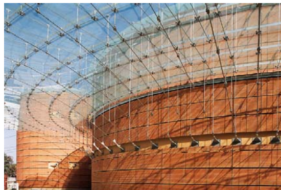
Dating back to 1887, Chartres cathedral (left) is a good example of the longevity of steel structures. Above, successful combination of steel with glass and wood (school at Ecully, in France), and with glass and brick (bank at Lodi, in northern Italy).
