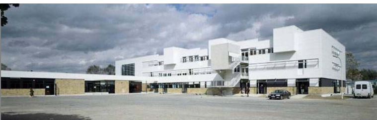
Before... after. The rehabilitation of Collège Pierre Corneille, in Tours, required only 3 months' work. It is a 1969 building, of which only the structure was retained. The facades were totally renovated with smooth pre-painted steel cladding installed on a subframe, and additional projecting volumes were created. Parts of the floors were deconstructed in order to produce a 3-storey concourse in the entrance area.
