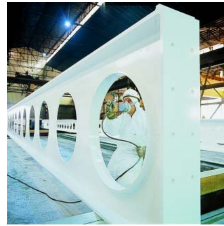
Steel frames are manufactured to very precise tolerances.
