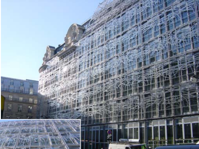
For the rehabilitation of the Ministry of Culture in Paris, Francis Soler devised a stainless steel mantilla that confers a common signature on the three disparate buildings that comprise the Ministry.
