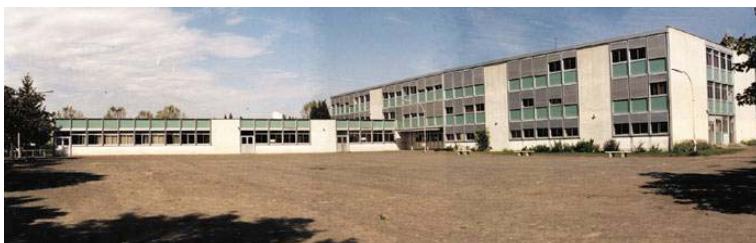
Before... after. The rehabilitation of Collège Pierre Corneille, in Tours, required only 3 months' work. It is a 1969 building, of which only the structure was retained. The facades were totally renovated with smooth pre-painted steel cladding installed on a subframe, and additional projecting volumes were created. Parts of the floors were deconstructed in order to produce a 3-storey concourse in the entrance area.
