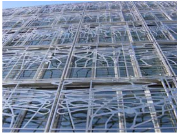
For the rehabilitation of the Ministry of Culture in Paris, Francis Soler devised a stainless steel mantilla that confers a common signature on the three disparate buildings that comprise the Ministry.
