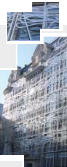
On the building's facade, the ornate stainless steel skin creates a calligraphic effect on the glass. An outstanding example of successful integration for steel.
