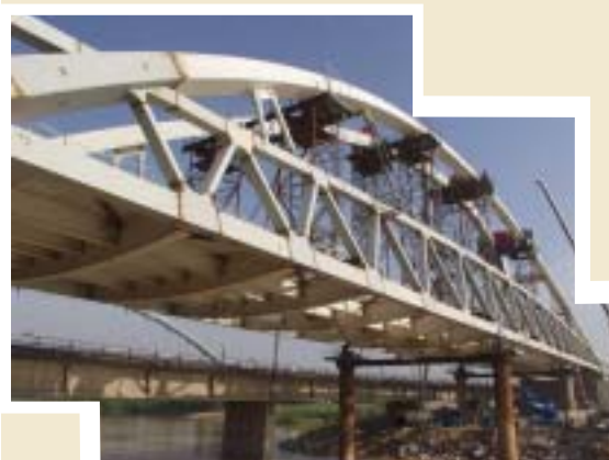
This very long span steel arch bridge, under construction in Zaragoza, illustrates the progress made by steel in HST bridges in Spain.
