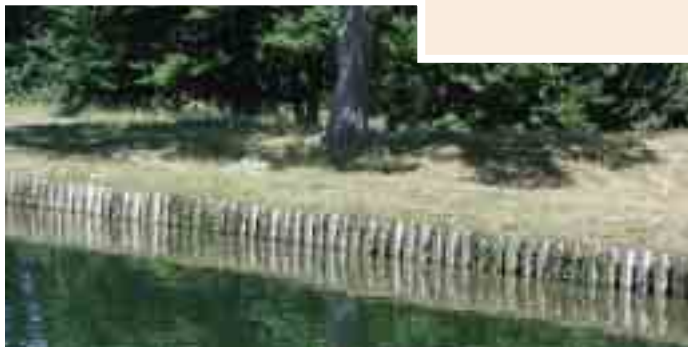
Employed for bank works, sheet piling retains the soil, thus facilitating the rooting of vegetation and encouraging fauna.
