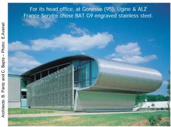
In the construction sector, stainless steel is employed above all for finishing works, roofcoverings and facades, and very rarely for structures. In other words, very little in the way of long products. When beams (which are generally welded plate sections) are employed for structures, they do not undergo any special preparation. As for tubes, they are generally polished, micro-pellet blasted, shotblasted.
