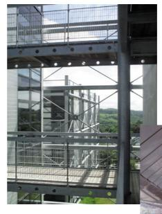
Apart from its corrosionresistant properties, bare galvanised steel is also employed for its attractive finish. Here for the structure and envelope of a business incubator in Cherbourg (left) and a motorway maintenance facility (below).
