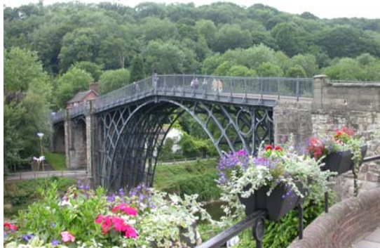
Figure 11 : Iron Bridge – Birmingham (1779)
